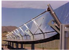
Figure 5. Parabolic Trough Collector
