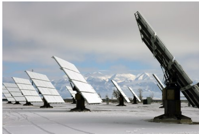
Figure 2. Solar Tracking PV Array
